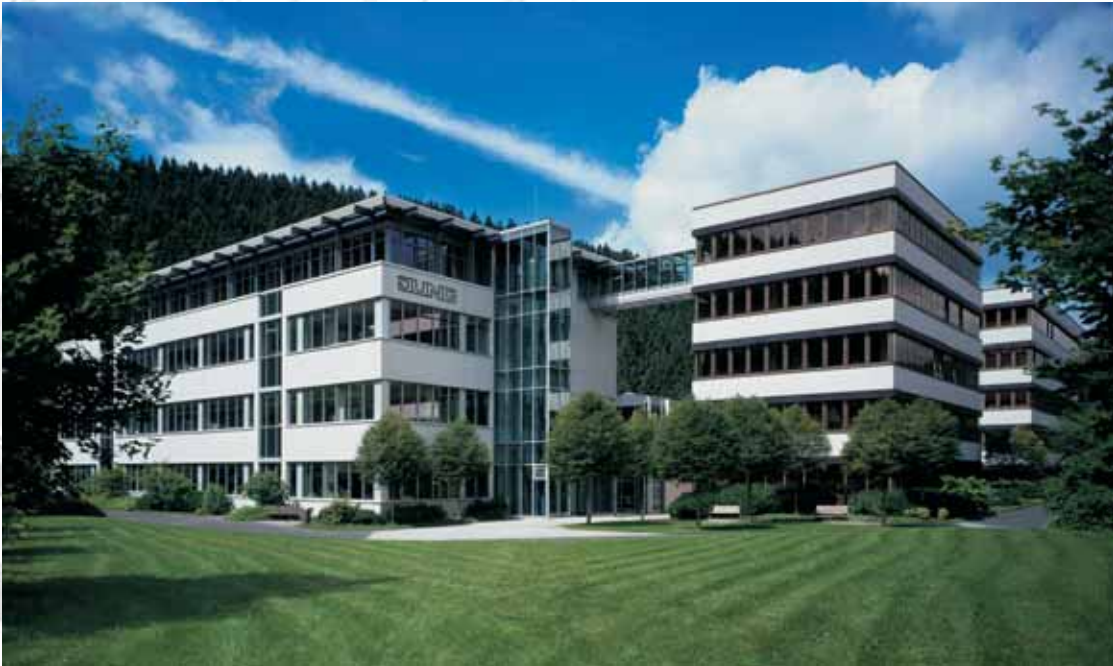
Administration, training centre and production in Schalksmühle
