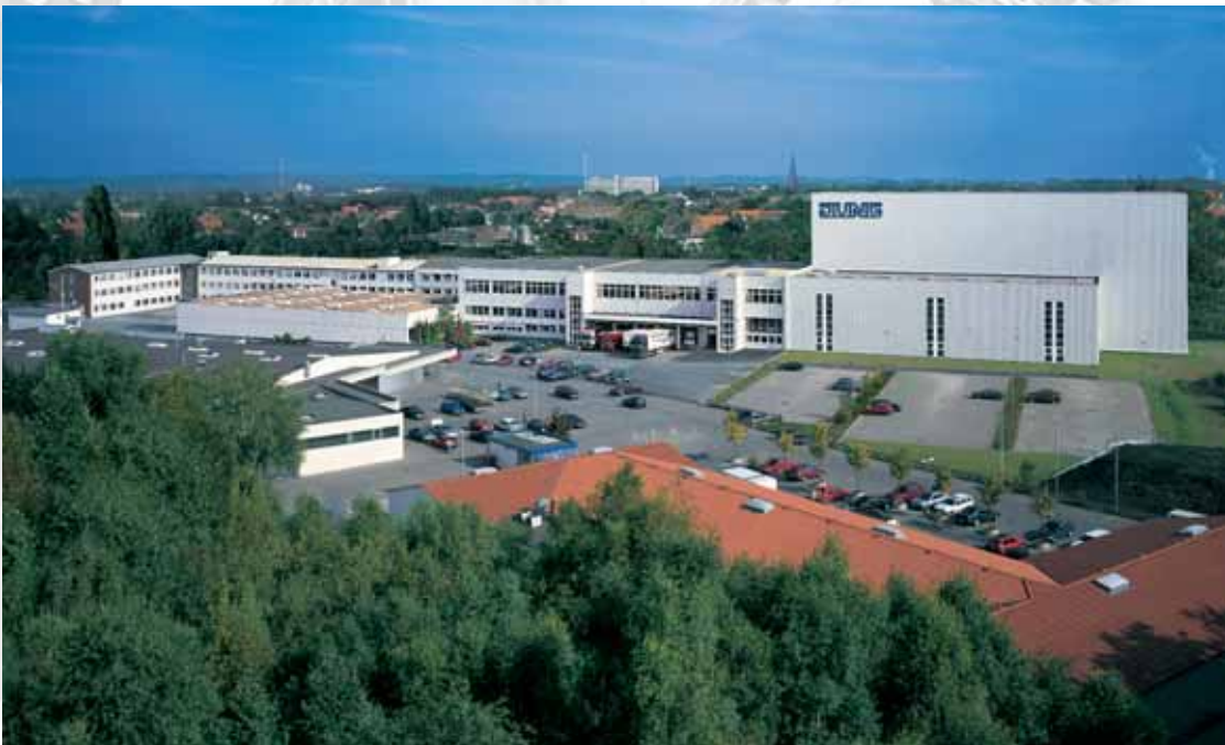
Production and high-bay warehouse in Lünen
